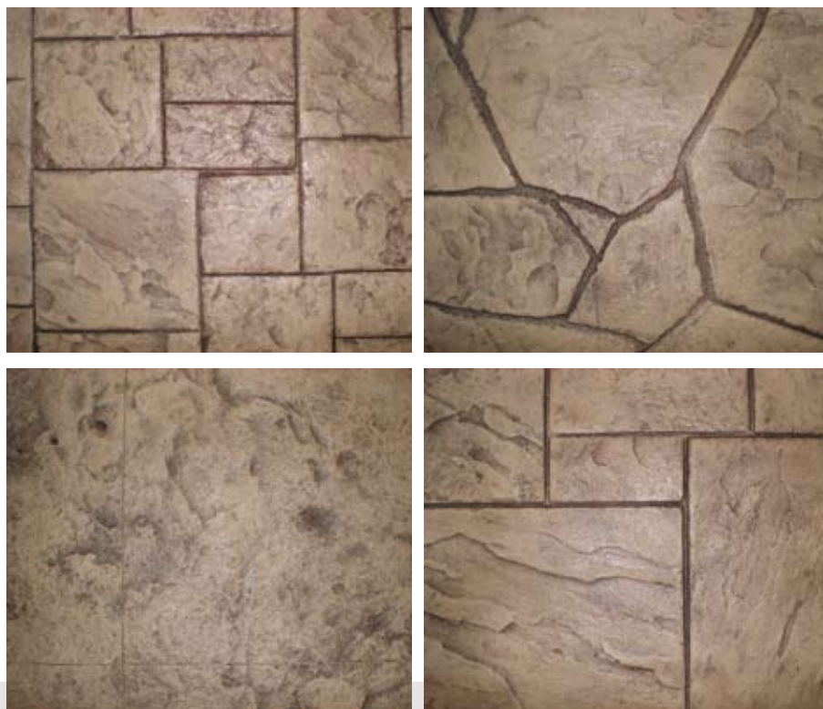
Popular concrete stamp styles: Top left: Ashler Slate pattern. Top Right: Random Flagstone pattern. Bottom right: Yorkstone pattern. Bottom left: Roman Slate pattern.
